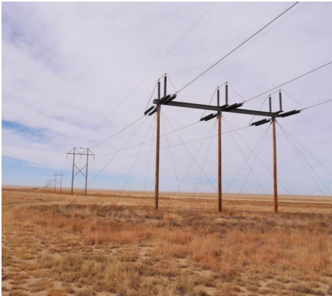
Tower #287 on the 230 kV transmission line crossing the property.
